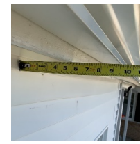
Soffit Depth
