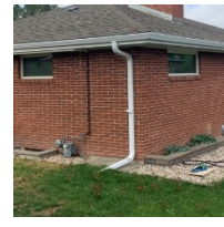
Full Downspouts (including Extensions)
