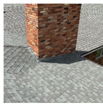
Chimney Flashings
