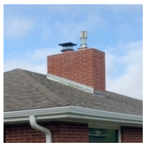
Counter Flashing
