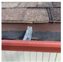
Gutter Fasteners
