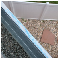
Gutter Damage
